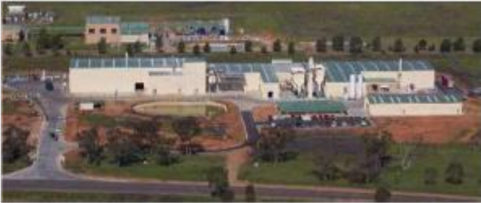
General Plant View
