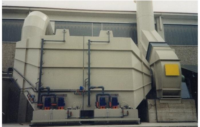
STC wet scrubbers are available in many configurations: horizontal, vertical tower, single, double or triple stages, venturi scrubber, fixed bed, floating bed.
